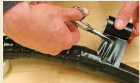
It is important that the ground kit be properly weather sealed. This bundled cable process provides labor savings and increased reliability. Composed of six rolls of Butyl Rubber tape and three rolls of black polyvinyl tape, the WK-U Weather Seal Kit provides everything necessary to properly seal one installed ground fixture.
